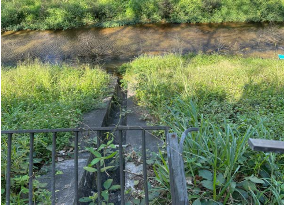
VIEW 5: Existing Final Discharge
